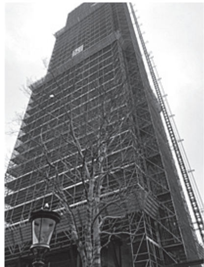
Dom Tower under restoration
